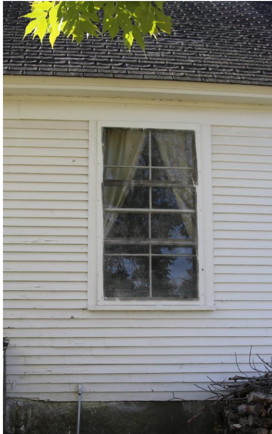
Photo 35: 4-over-4 window on the north side, recently restored, with wood-framed screen affixed to the exterior.
