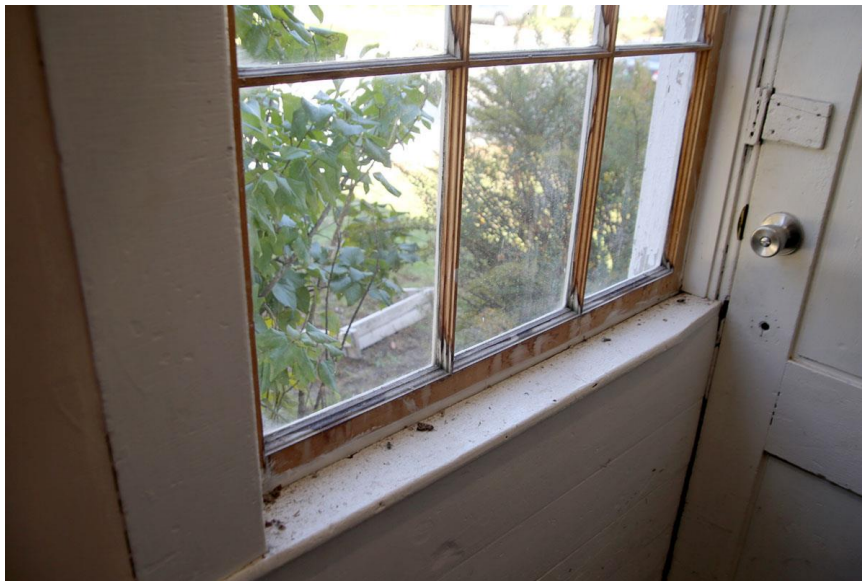
Photo 48: Interior of the 6-over-6 window on the west façade, showing water and UV damage.
