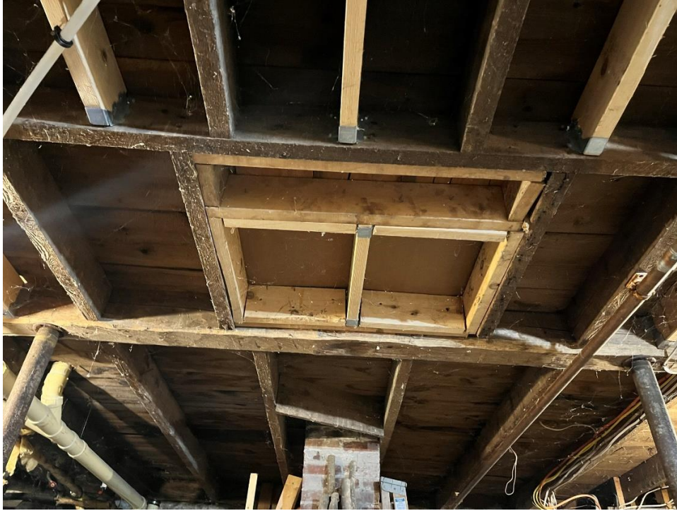
Photo 3: Evidence of an early central chimney in the floor framing, with the existing stove chimney behind
