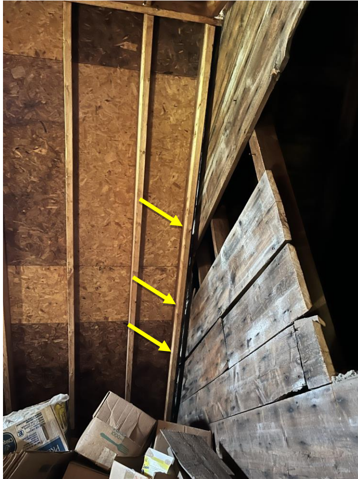
Photo 53: Gaps seen between the framing of the roof addition and the older building's east elevation (arrows)
