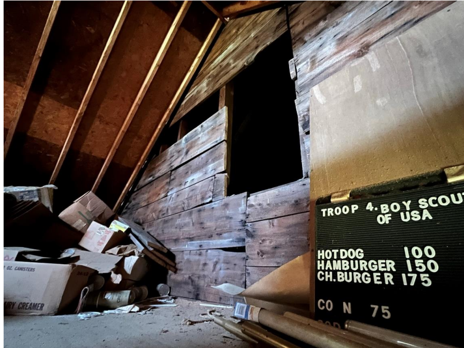
Photo 23: Roof rafters and plywood sheathing in rear addition and exterior sheathing of main building, east elevation.
