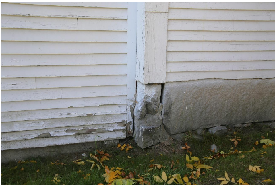
Photo 39: Northeast corner foundation, showing open joints and loss of mortar. Rot in the lower clapboards at left.
