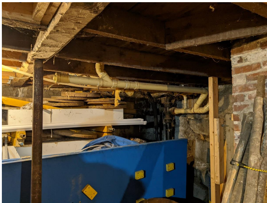
Photo 27: Handhewn main floor beam, above left, and waste line, chimney to the right (Flynn)
