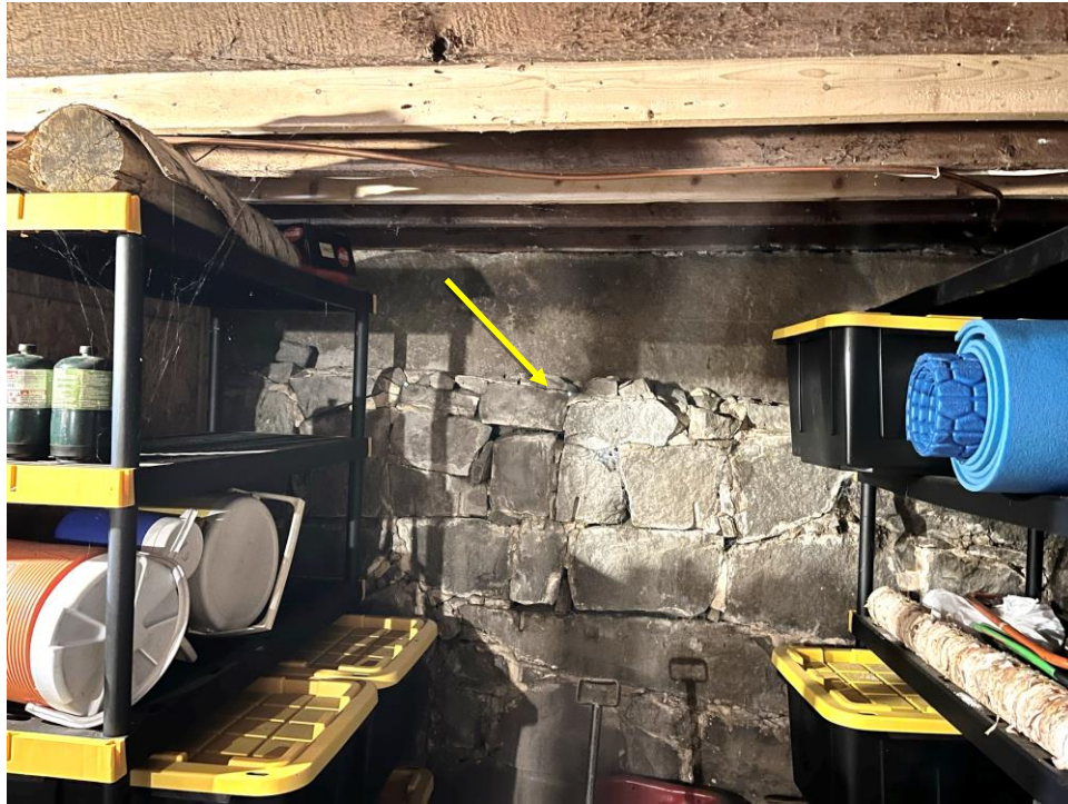
Photo 54: Granite foundation wall, north wall, showing loss of mortar and several areas of light shining through from the exterior (shown with arrow)
