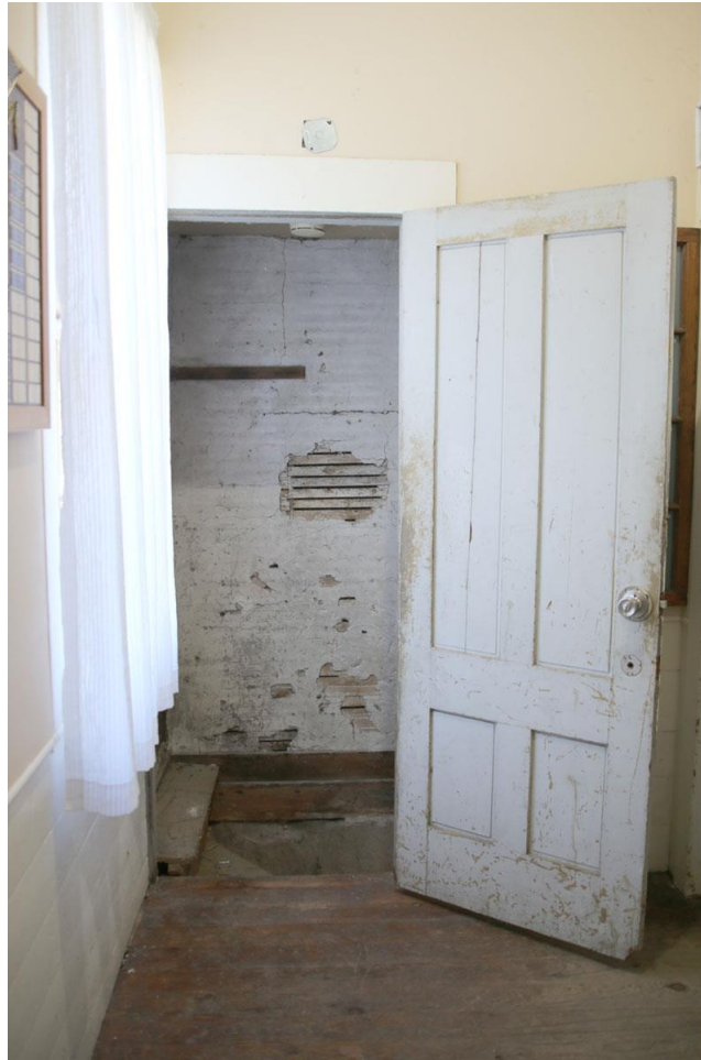
Photo 43: Doorway in lobby to the basement stairs, showing unfinished plaster on lath. Door likely dates to before 1900, around the time the building was relocated.
