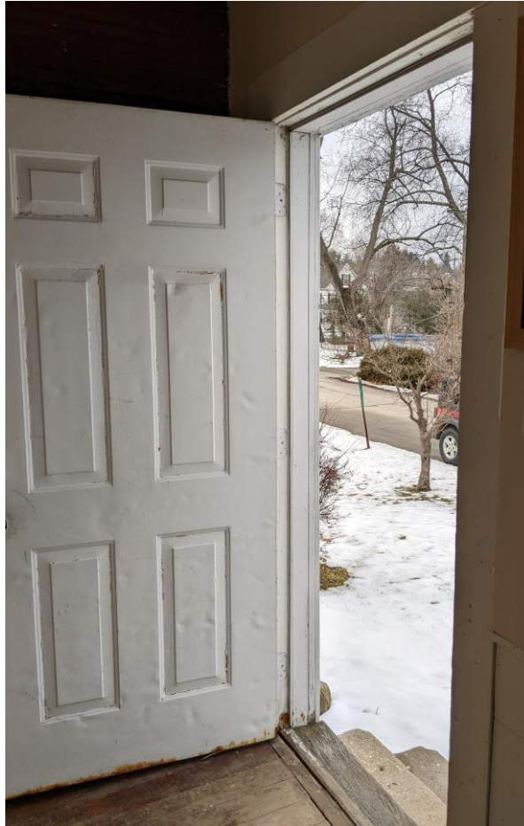
Photo 37: Front door, showing the dents in the surface and rust forming along the bottom edge (Flynn).
