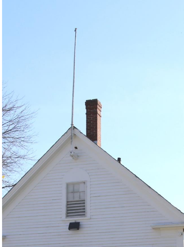
Photo 33: Flagpole and hole just beneath the peak of the gable on the façade.
