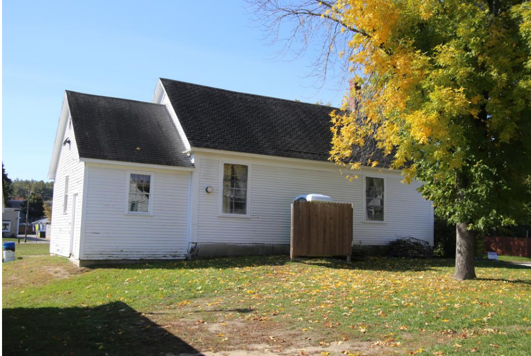
Photo 9: North elevation of the building, showing two 4-over-4 windows in the main building and a smaller 6-over-6 window in the addition.
