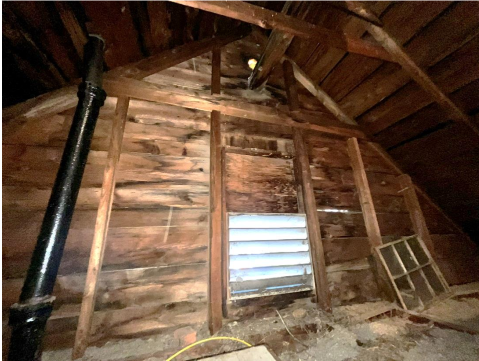
Photo 51: Attic interior, west (front) elevation of main building, louvered vent installed in the lower sash opening, with sash stored to the right.
