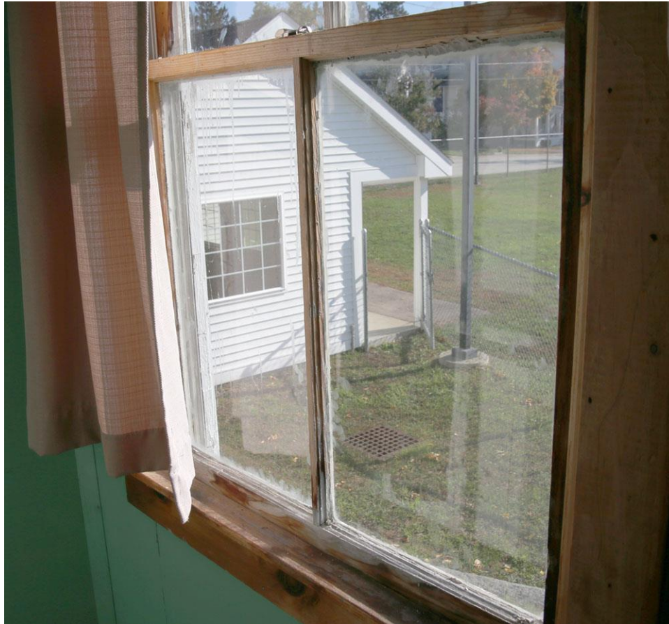
Photo 49: Interior of the 2-over-2 sash, showing deterioration of the wood and sill.
