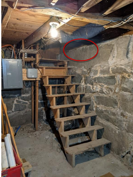
Photo 24: Original granite foundation with marks (pre-1830) laid on top of irregular cut granite scrap (Flynn)
