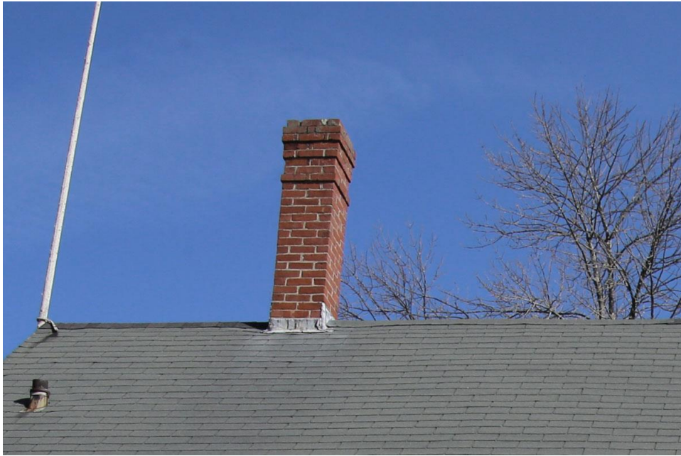
Photo 38: Brick stove chimney, with a few areas in need of repointing in the top corbeled section.
