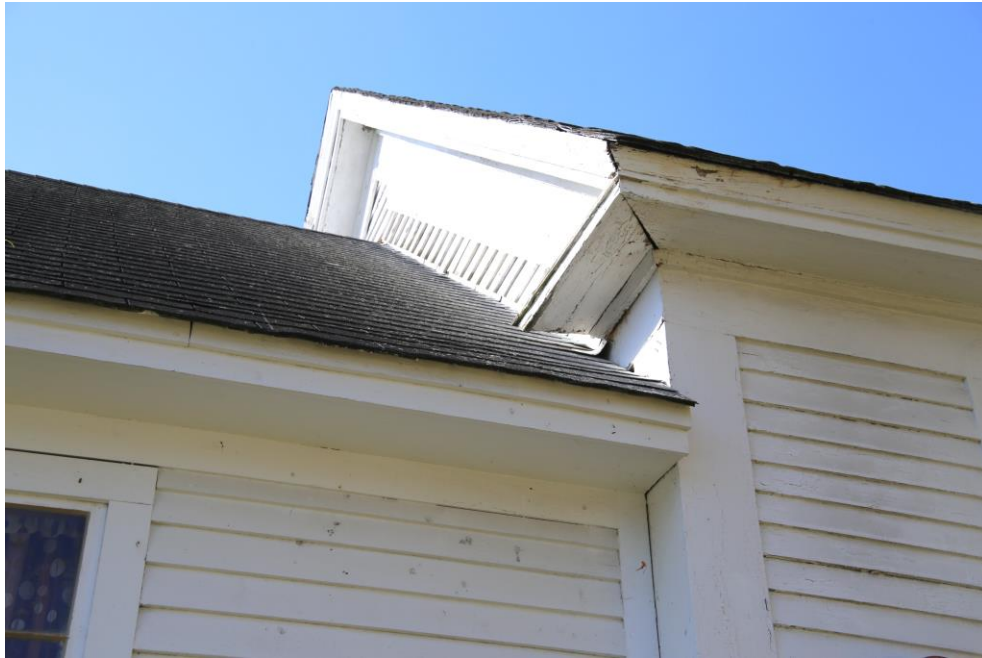
Photo 32: Cornice return on the northeast corner of the main building shows paint loss and open joints.
