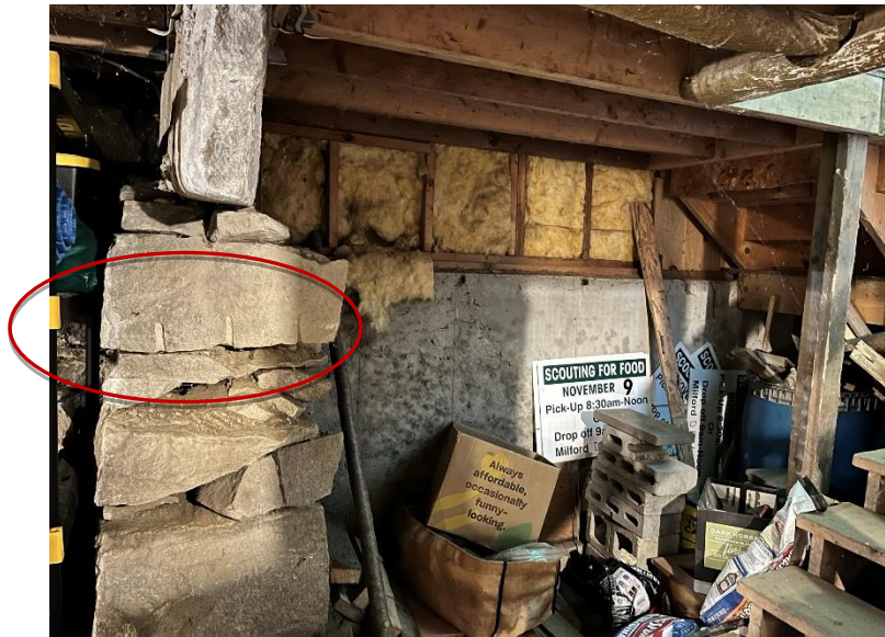
Photo 25: Granite block support with plug and feather chiseling (post-1830) and concrete foundation under rear addition (at right).
