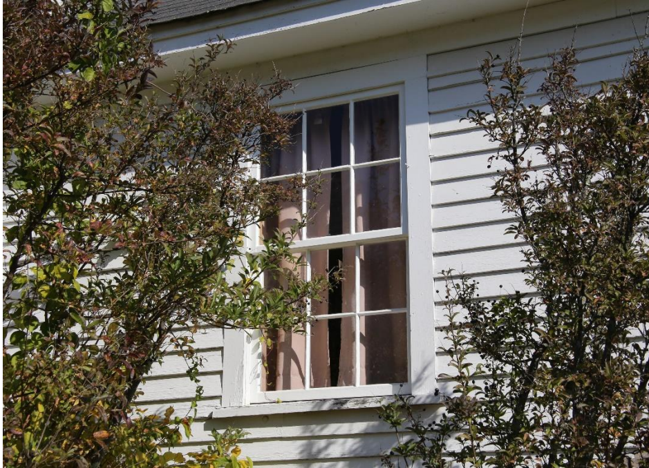
Photo 36: 6-over-6 window on the south side of the addition.
