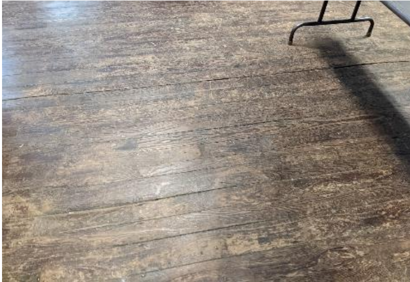
Photo 44: The flooring in the main room is slightly uneven due to age and use but is in good condition (Flynn).
