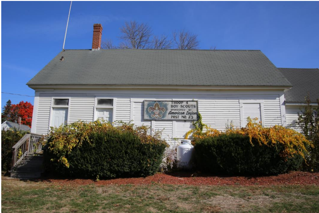
Photo 29: South elevation showing roof, closed window openings, and vegetation growing close to the exterior wall.
