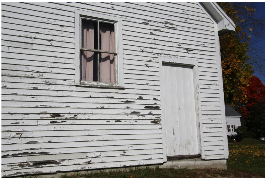
Photo 31: East elevation, part of the 1980s addition, showing severe loss of paint on the wood trim and clapboards. The 2/2 window is an older window reused in the construction.
