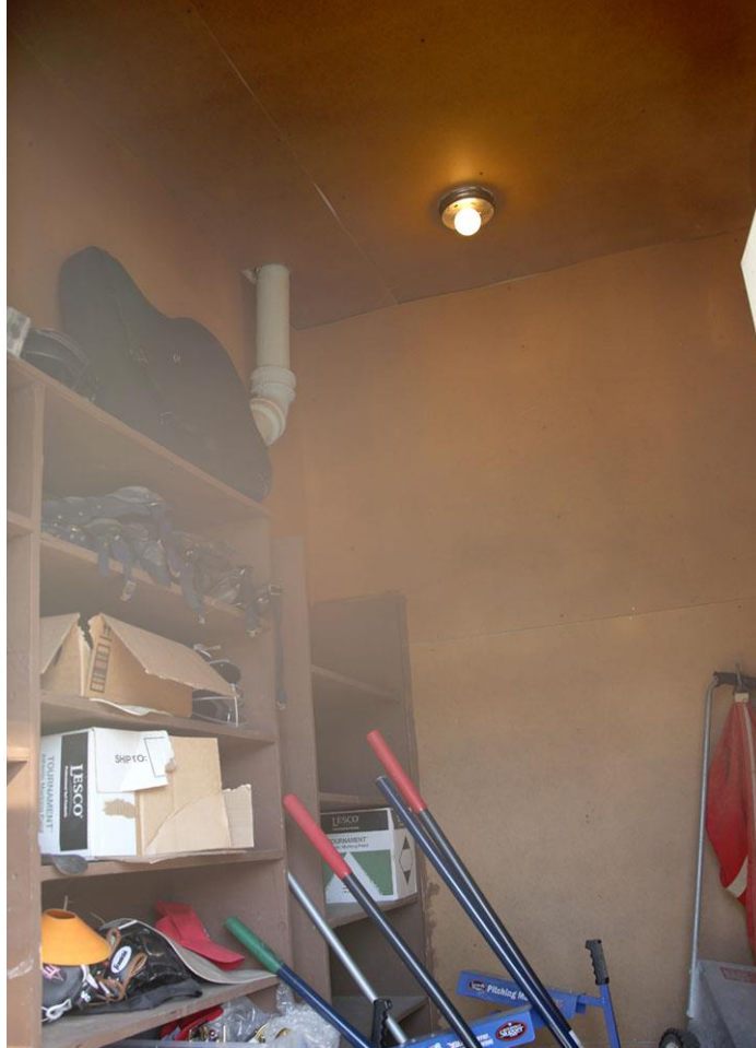
Photo 46: Interior of the storage room, showing MDF panels applied on the surface of the walls and ceiling. Cast iron vent pipe seen at upper left.
