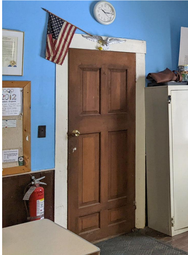
Photo 50: Door between the lobby and the main room is in good condition but has been hung upside down, making the knob height high.
