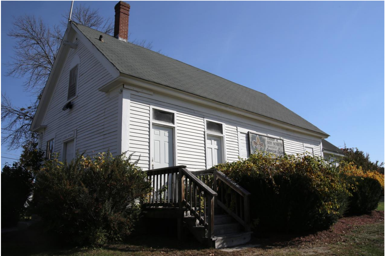
Photo 5: The roof is asphalt shingled with an interior chimney and plumbing vent in the southwest corner.
