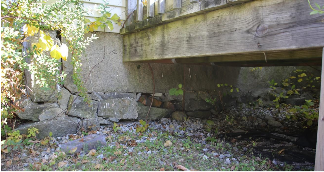
Photo 40: Southwest corner foundation, showing loose stones and open joints. Stair landing to storage room at right.
