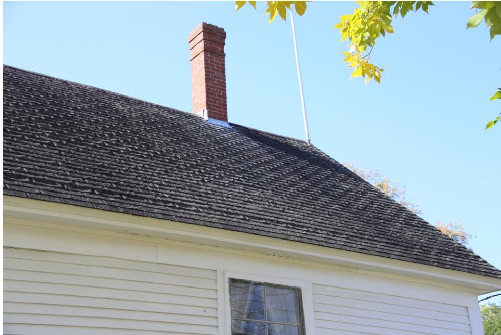
Photo 30: North elevation roof, showing degradation and curling of the asphalt shingles.
