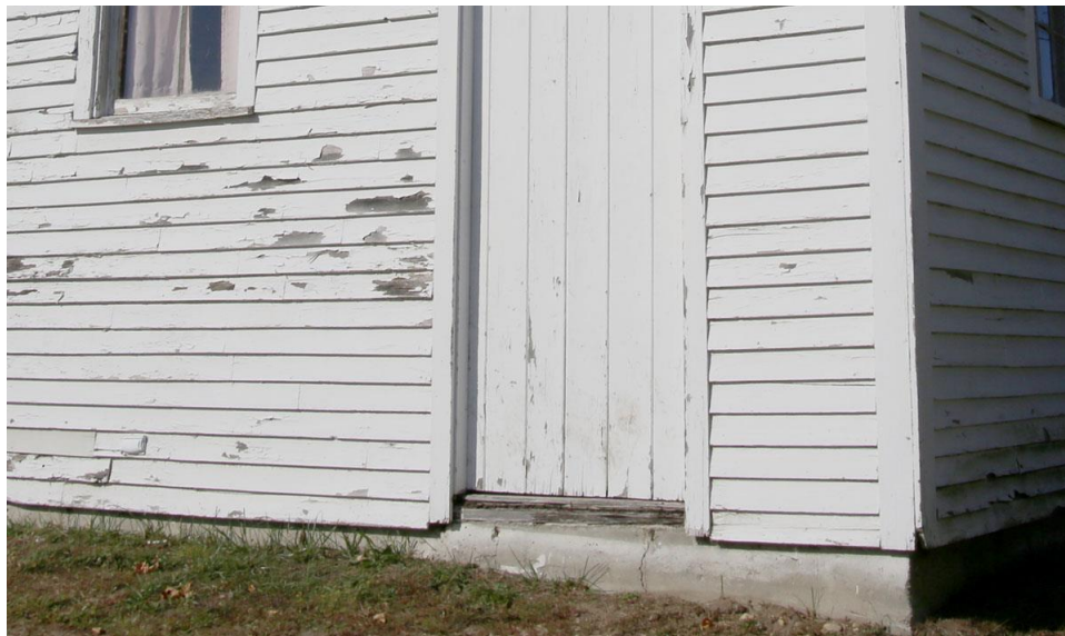
Photo 42: Cracks seen in the concrete foundation beneath the deteriorated door sill on the east elevation.
