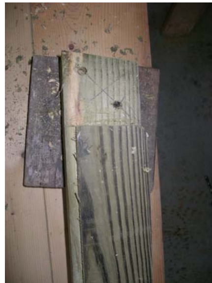
Photo 2-4: Location of holes for lag screws
