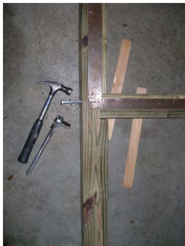
Photo 2-5: Facing edges shimmed before vertical and cross members are joined with lag
